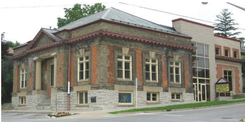
Existing Paris Branch Library at 12 Williams Street
